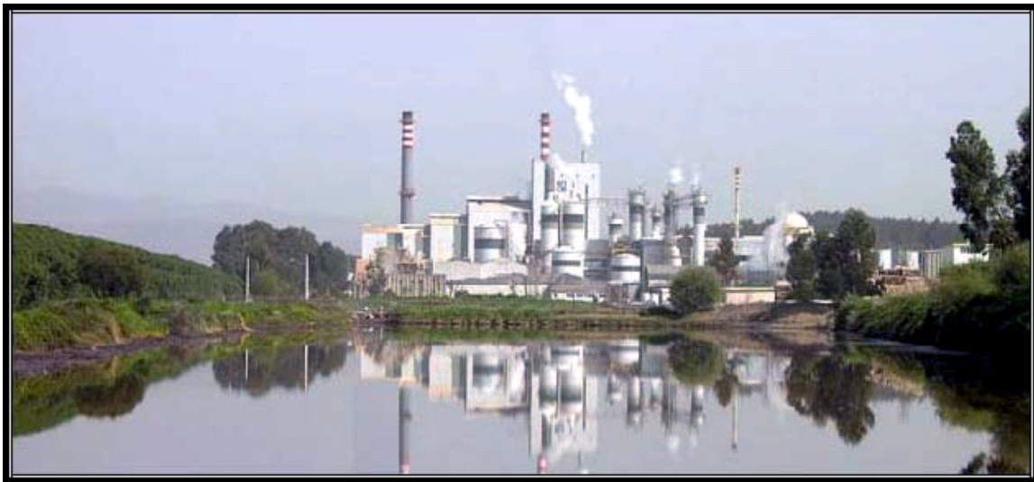
Figure 1.1-6: Example of ENCE Mill Operation in Spain
